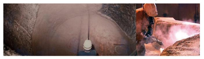
Magnesia based refractories (basic refractories) have the ability to withstand high temperatures, show high resistance to basic slags and sufficient strength to withstand mechanical abuse and abrasion in hot environments. Also where steel cleanliness is of the highest importance, basic refractories are recommended.
